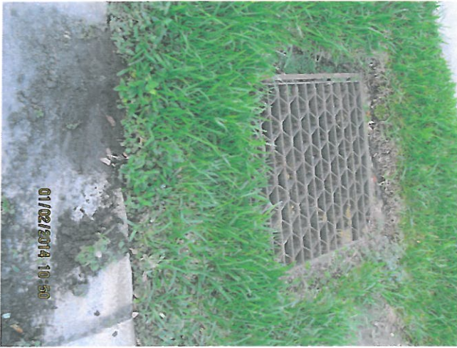
Typical inlet in grassed area East Side
